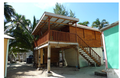
4. Tobacco Caye Marine Station completed
