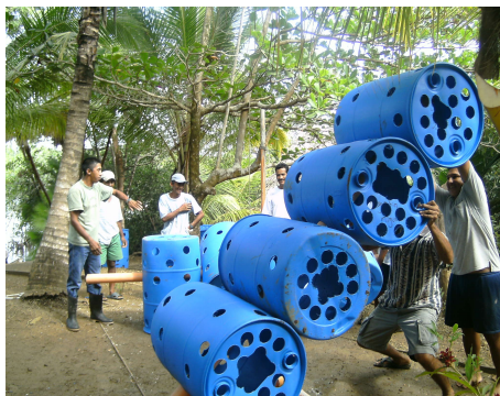
5. Fishermen building the fish aggregators
